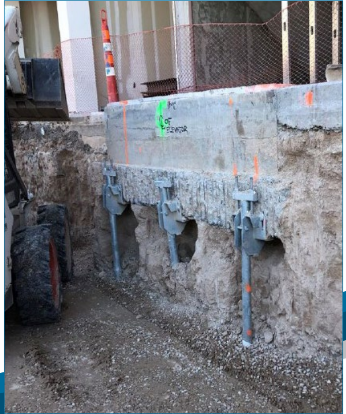
Exposed vertical cut helical piers. The soil here was treated with SoiLok.
