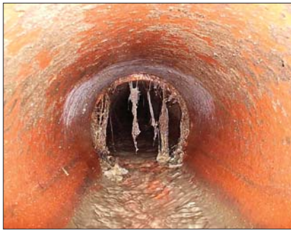
Common manhole problems: Above, roots growing in the pipe joint; below, roots growing in from the wall and pipe seal.
