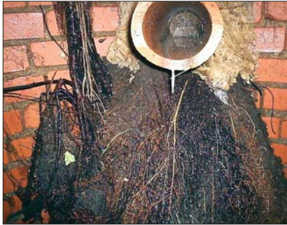
Common manhole problems: Above, roots growing in the pipe joint; below, roots growing in from the wall and pipe seal.
