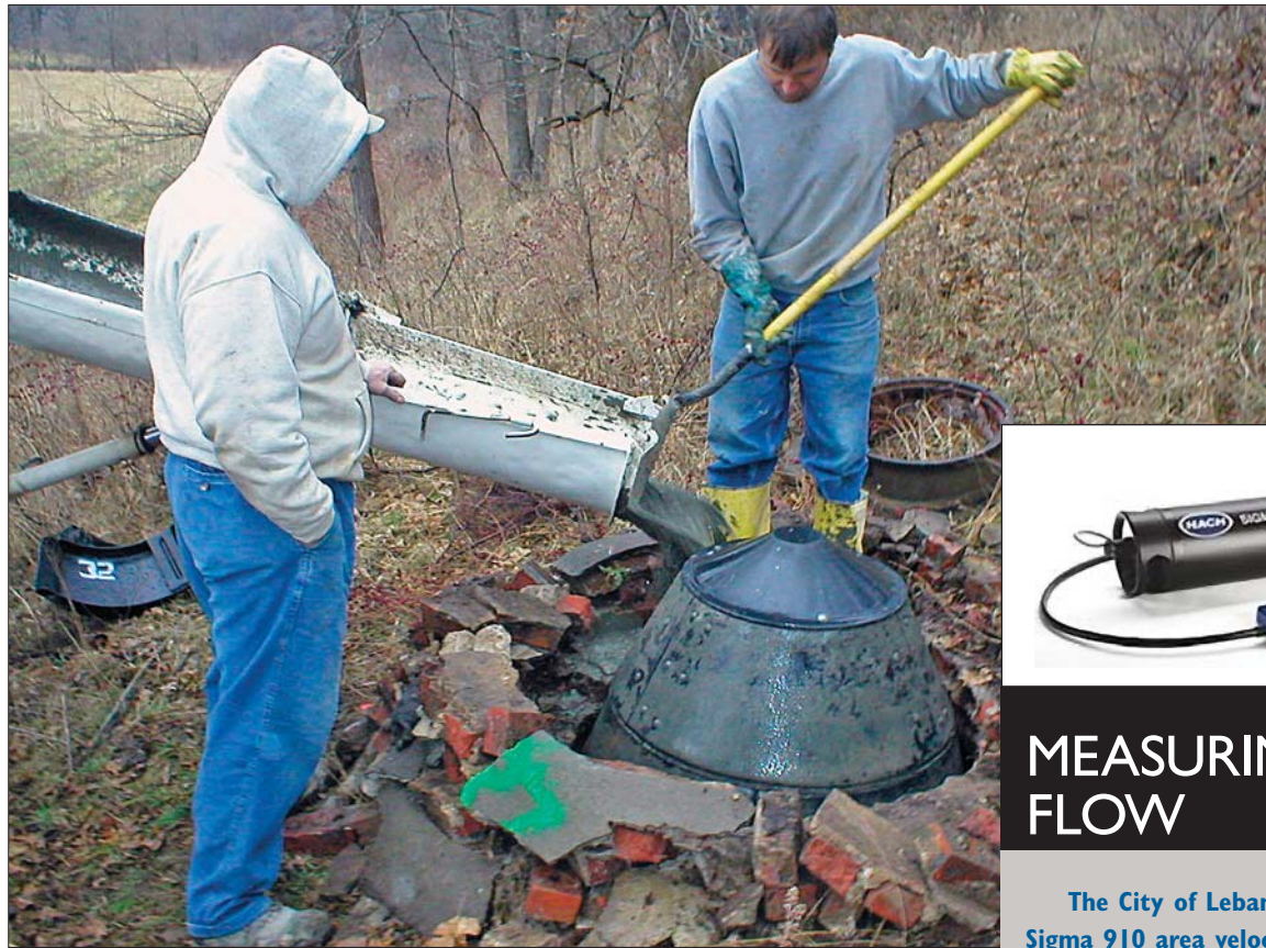
A technician pours concrete into forms inside an existing manhole.
